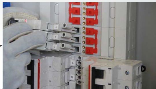
The Breaker Is Inserted Into The Opening
