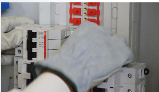
The Breaker Snaps Into The DIN Rail
